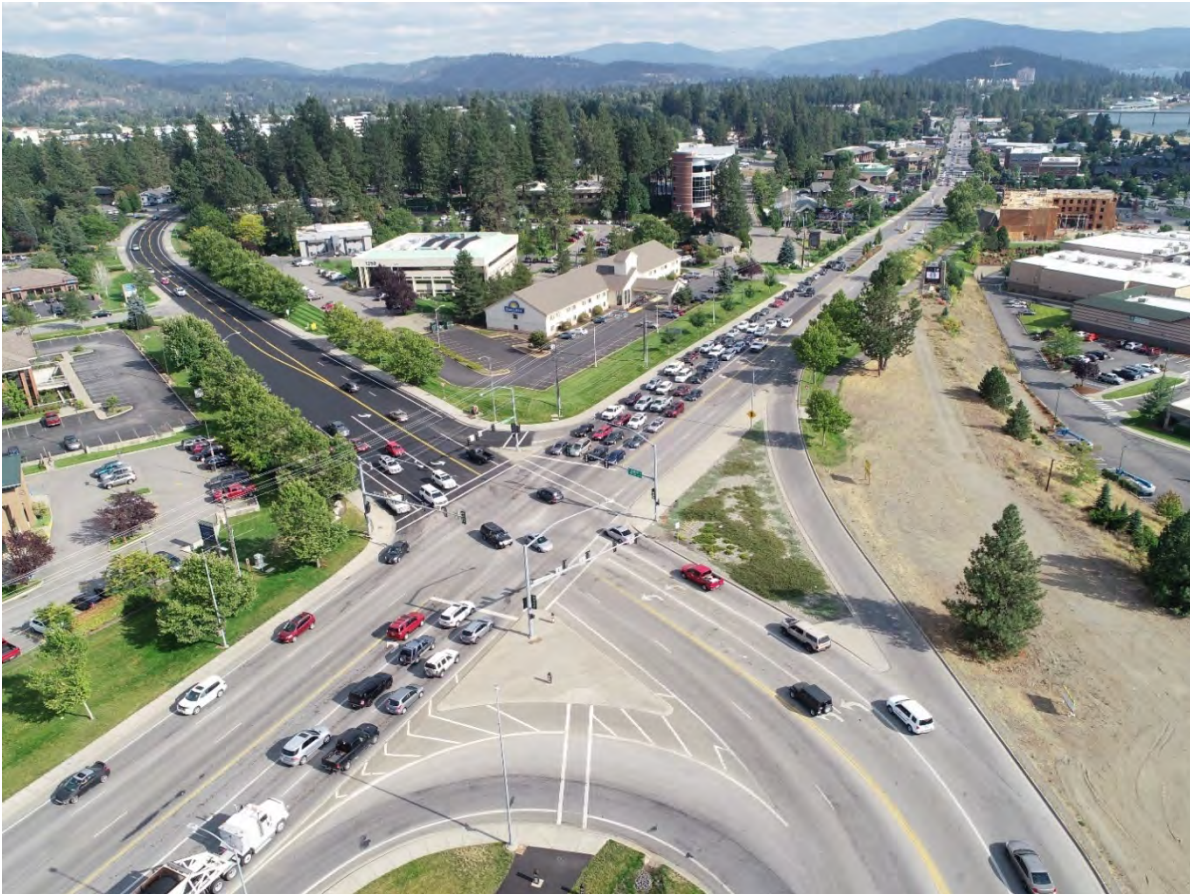
Figure 10-1: Intersection of Northwest Boulevard, Ironwood Ave, and Seltice Way looking southeast
